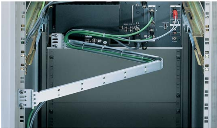
Cable support without return spring
