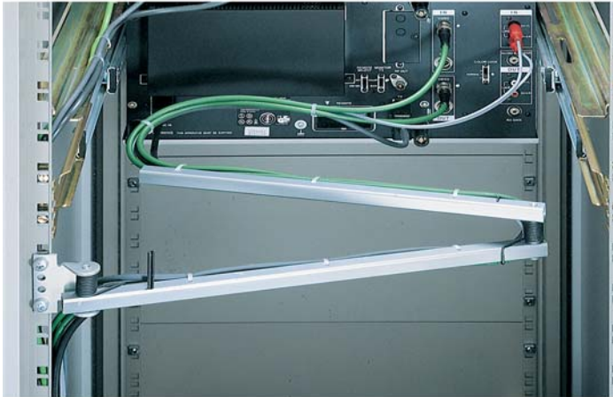
Cable support with return spring
