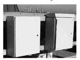
Hoffman's research of the effects of solar radiation on enclosures has shown the positive benifits of utilizing shielding to decrease temperature rise. Shielding has been found to be an effective, low-cost method of reducing solar heat gain in outdoor electrical/electronic applications.
